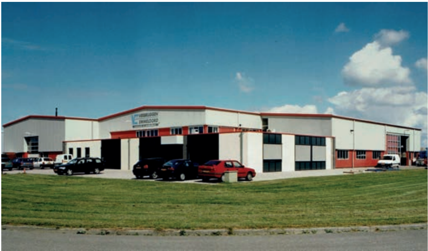
New accommodation at the Dukaat
